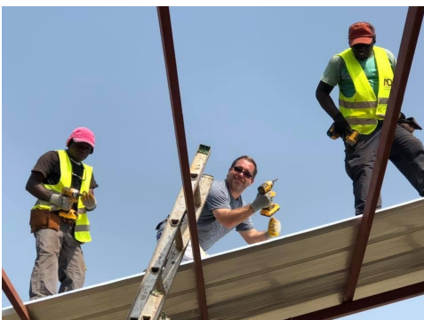
(Jeff Stender drilling sheet metal with IC team)
